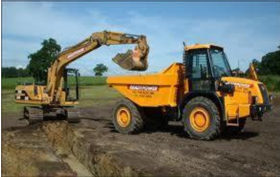
EXCAVATOR AND DUMP TRUCK
